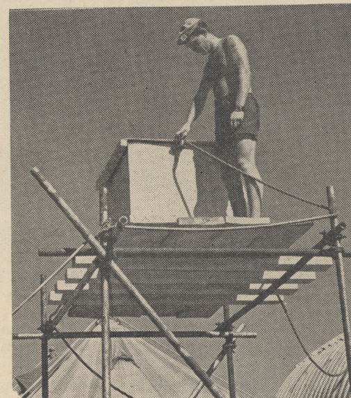
Cpl Bob Wilkinson, who is with men of the Anti-Tank Platoon at Anadhiu, controls the tank water level on top of the newly constructed 'tower'.
